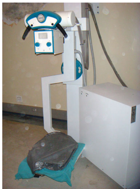
Fig. 3 A WHIS-RAD unit at a World Health Imaging Alliance (WHIA) site in South Africa, which had to be protected after a fire broke out in the room endangering the equipment
